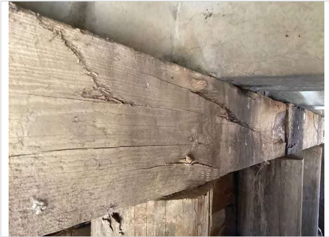
Abutment 1 cap splintered areas and grain checks up to 1/16"
