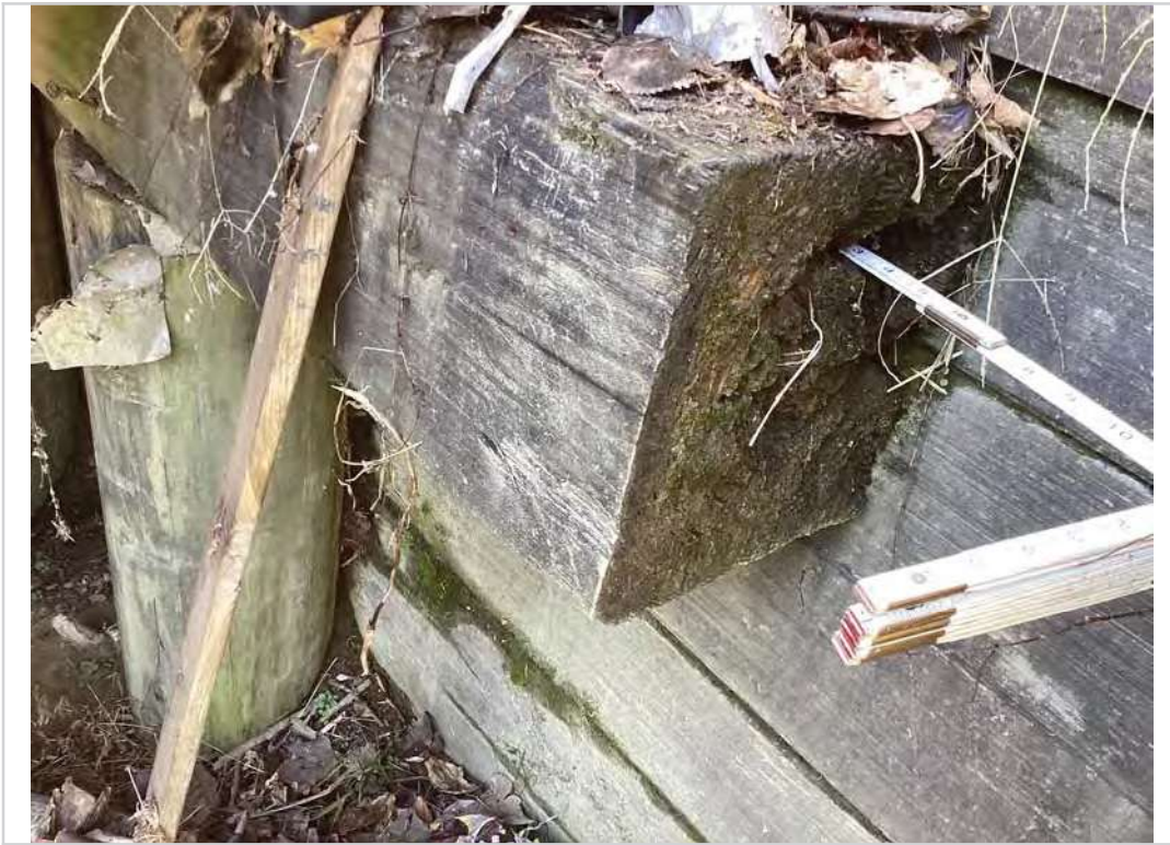
Abutment cap 1 left end decay
