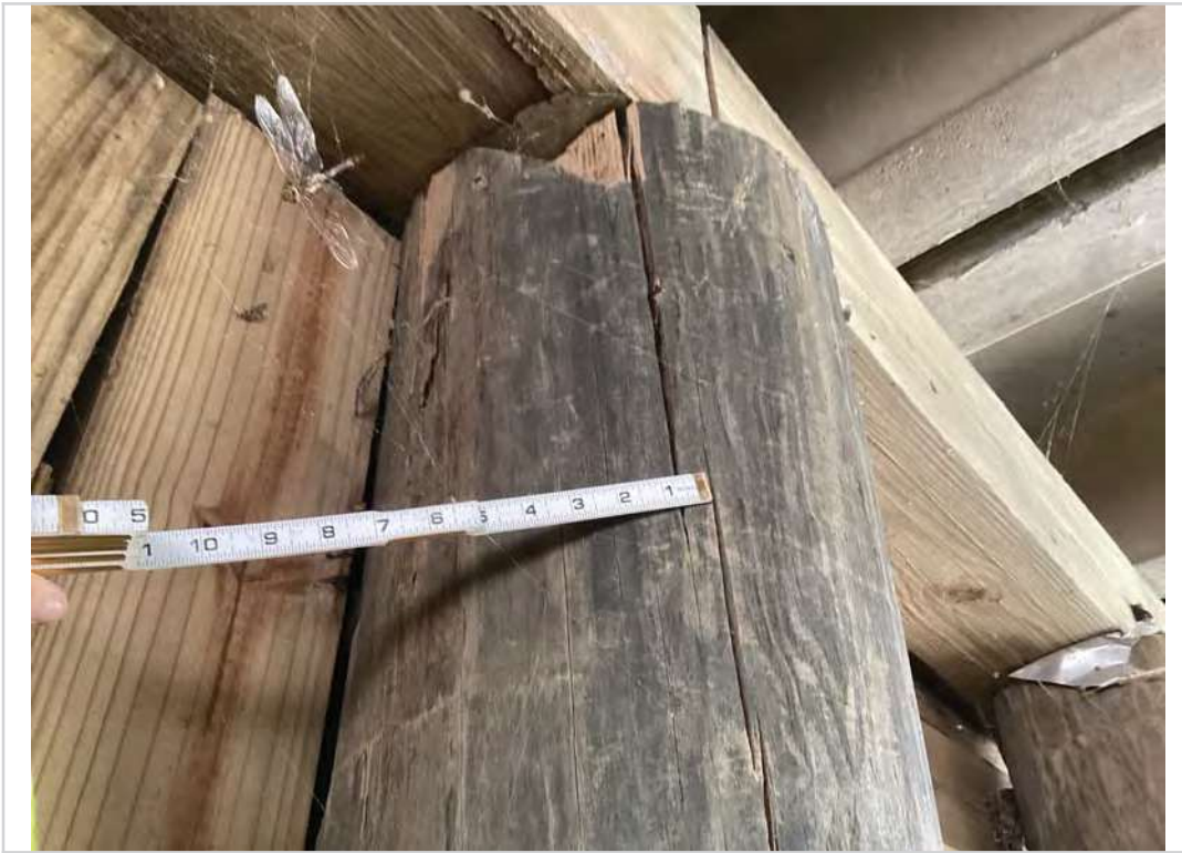
Abutment 2 pile "F" 1/2" check
