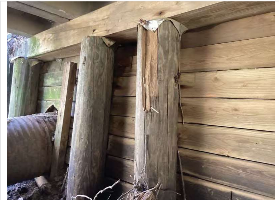
Abutment 2 pile "C" splintering
