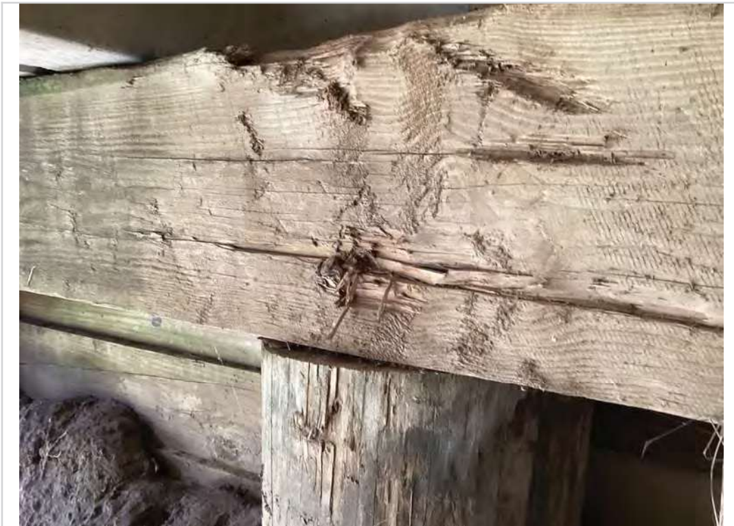
Abutment 1 cap splintered areas and grain checks up to 1/32"
